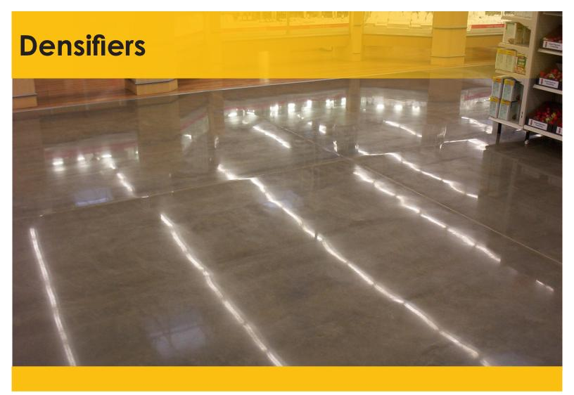
7937, Concrete Densifier is a one component water based, lithium based designed to densify cement and concrete. The lithium based densifier reacts with the cementitious ingredients to densify while allowing deep penetration to chemically harden and fortify the substrate.
