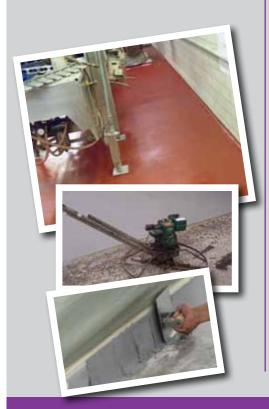
Epoxy Mortar is a heavy duty, troweled floor topping that can be used to patch or resurface concrete and cement floors. It is composed of a unique blend of aggregates and polymer resins. These products offer superior durability and resistance to heavy traffic.
