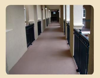
Additionally, the use of the aggregate allows slip resistance for both pedestrian and vehicular traffic.
